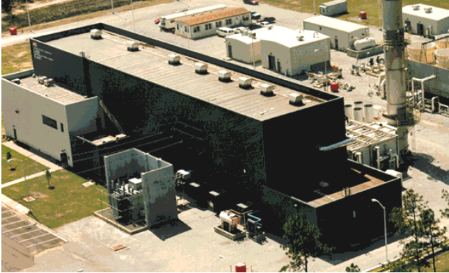
Alabama Electric Cooperative's CAES Plant (110 MW-26 Hr).
